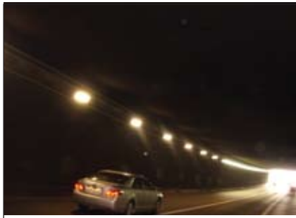
Korea Daqui Tunnel
